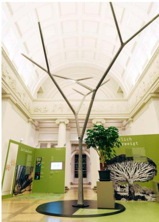
Fig. 3: Branched supporting column with braided textile hull consisting of carbon and glass fibers inspired by the outer form and structure of the branching regions of *Dracaena marginata* and *Schefflera arboricola* and developed in the A06-project at the TRR 141 exhibition in the State Museum of Natural History in Stuttgart. This demonstrator will find its final home in the entrance hall of the FIT building in Freiburg. © PBG & SMNS
