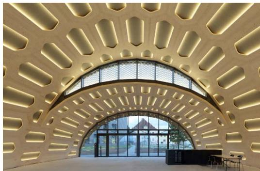
**Fig. 4:** Interior of the *livMatS* Biomimetic Shell @ FIT showing the solar gate weather-sensitive shading system. © ICD/ITKE/IntCDC University of Stuttgart, Photo: Conné van d'Grachten
