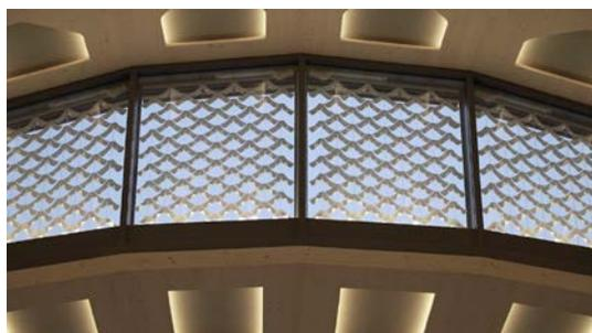
**Fig. 5:** Solar gate weather-sensitive shading system. © ICD/ITKE/IntCDC University of Stuttgart, Photo: Conné van d'Grachten
