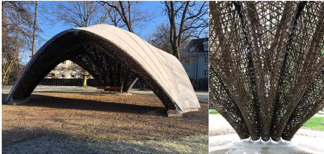
Fig. 2: Winter view of the cactus wood inspired sustainable "livMatS Pavilion" in the Botanic Garden Freiburg and details of the reticulated supporting structure. © Plant Biomechanics Group Freiburg. Detailed information may be found at the following link.
